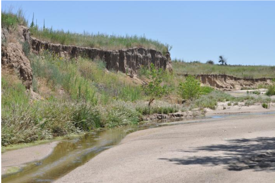
Photo 9: Looking east along Coal Creek at the fringe wetland abutting the creek on the north side and vertical eroded banks of Coal Creek (Wetland CCC).
